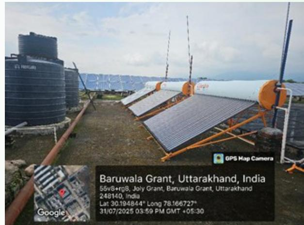
The University has also installed a 50,000 LPD solar water heating system, supplying round-the-clock hot water to hospital wards and hostels. Over three years, this system has offset approximately 22.5 lakh kWh of electricity consumption, delivering substantial energy and cost savings while supporting critical healthcare operations.
