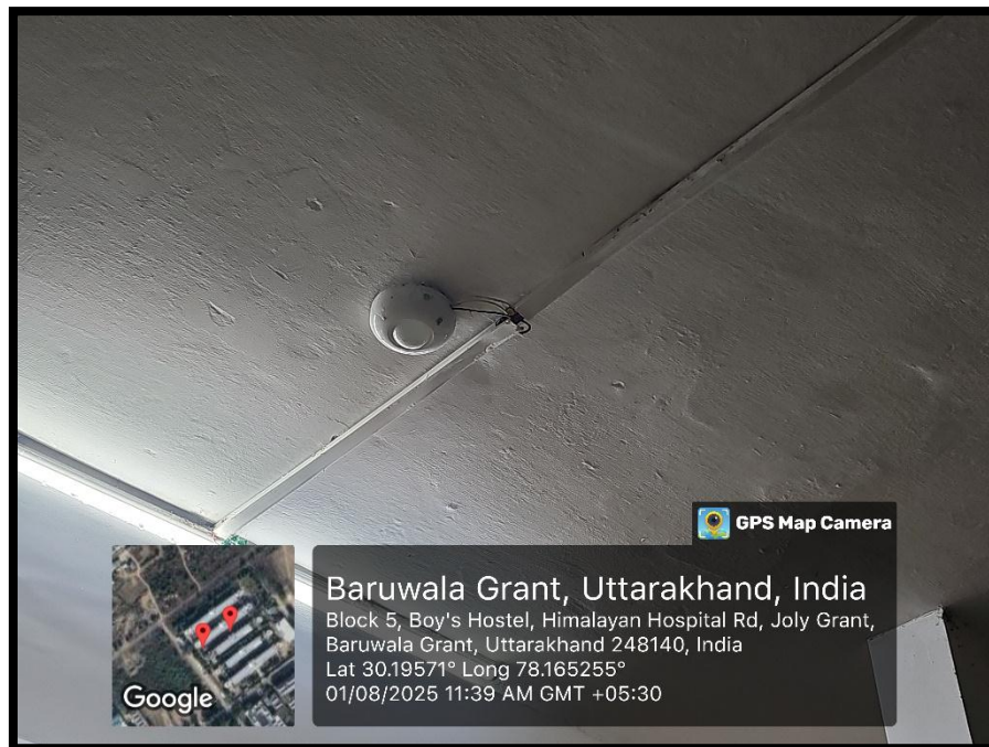
Picture: 3: Motion Sensor for Lights
