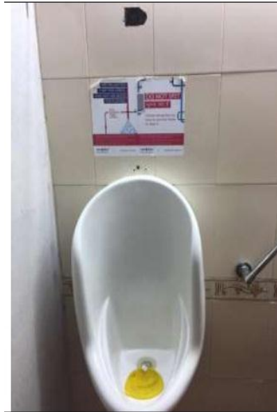
Figure 3.4. Waterless urinals (200 Nos.)
