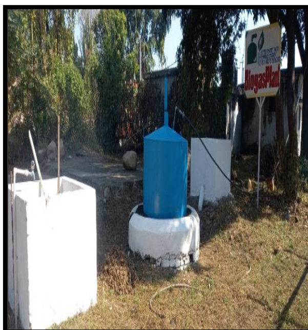
Figure 7.4. Bio-gas Plant of capacity 4 cum/day
