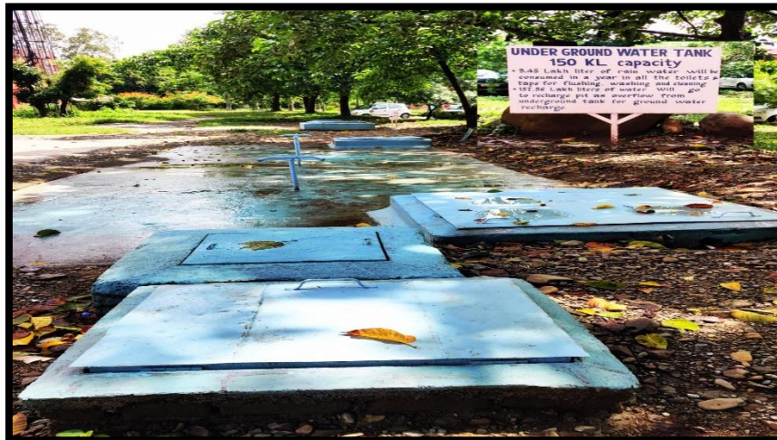
Figure 3.3. Underground water tank of 150 KL capacity
