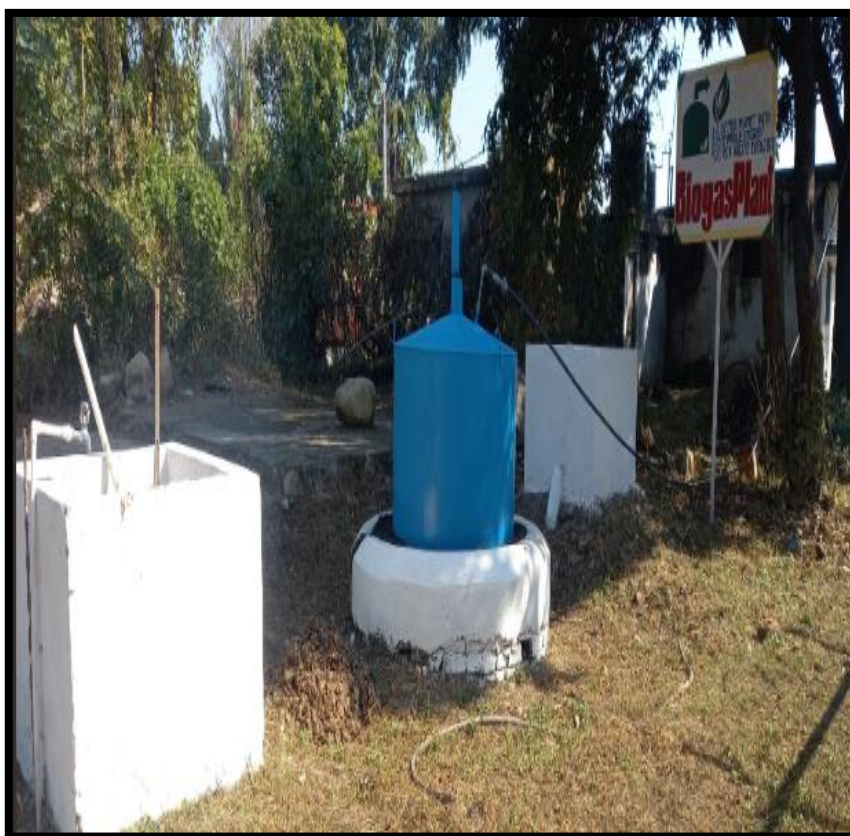
Figure 4.1. Bio-gas Plant of capacity 4 cum/day
