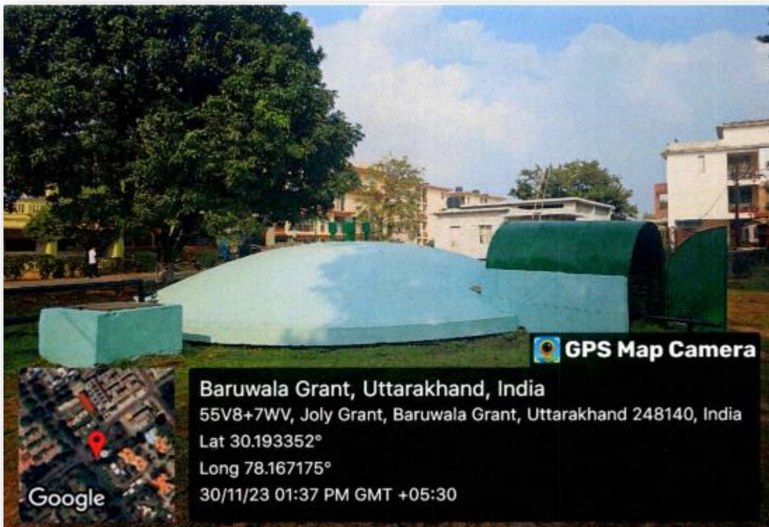
Distribution pipe from the tubewell to underground well
