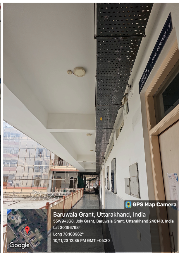
Motion based sensor lights at HSST building
