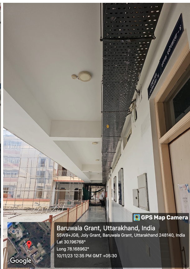
Motion based sensor lights at HSST building
