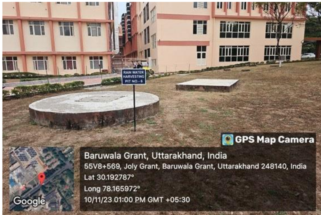
Rain-Water Harvesting Pit
