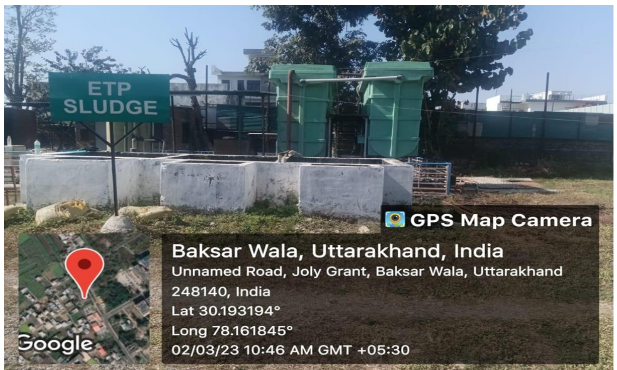
Effluent Treatment Plant
