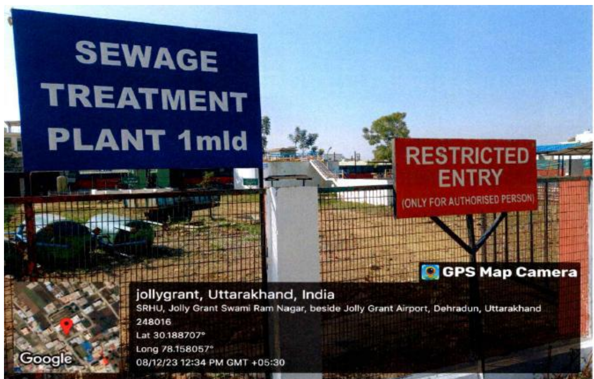
Sewage Treatment Plant
