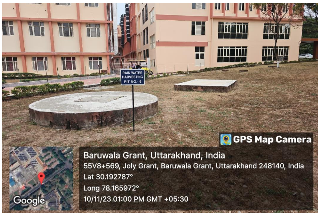
Rainwater harvesting pits with filter bed recharge near Cardiac OPD building
