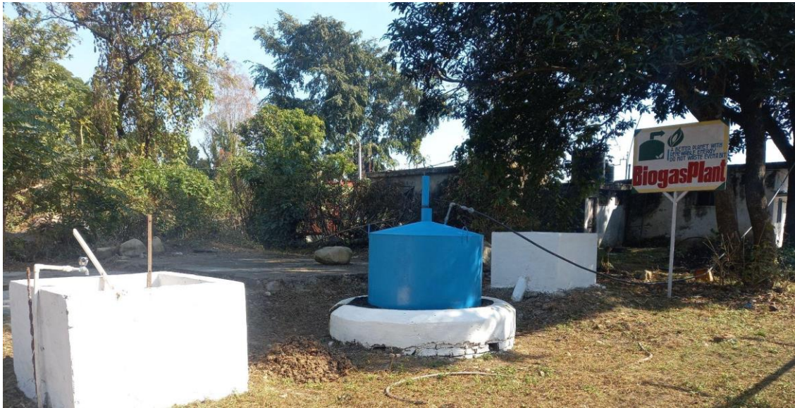
Biogas plant at Swami Rama Himalayan University converting organic waste into clean cooking fuel
