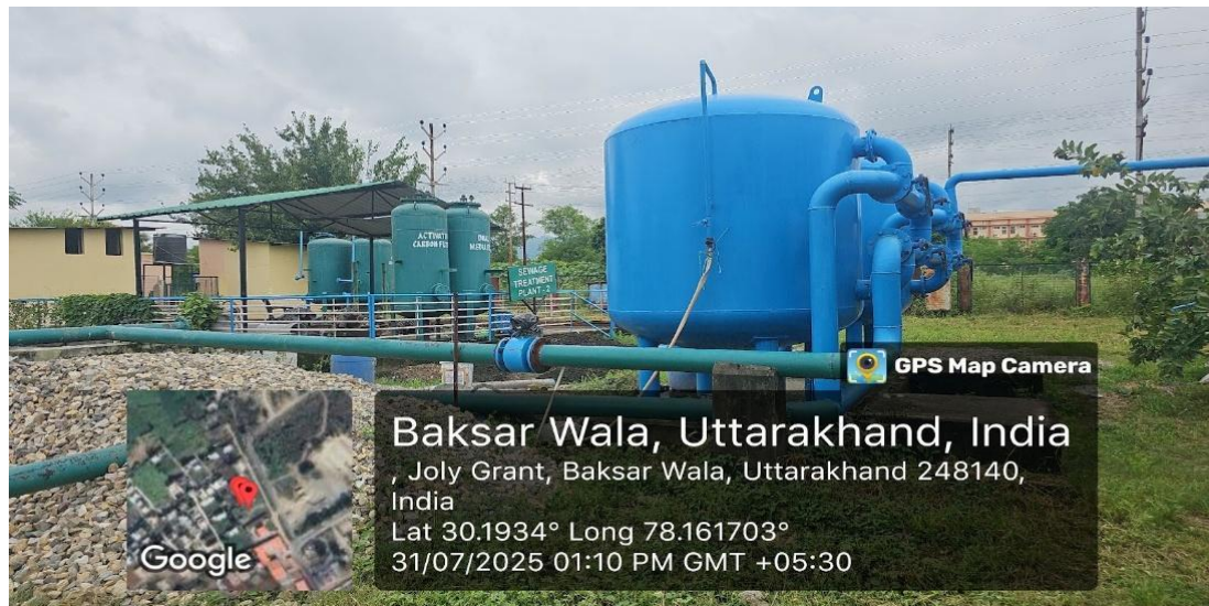
Sewage Treatment Plant at the University
