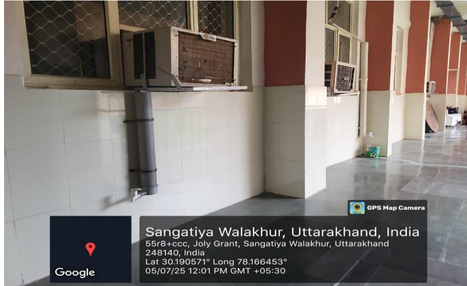
Condensed water from AC Units is used across the campus to repurpose and recycle water
