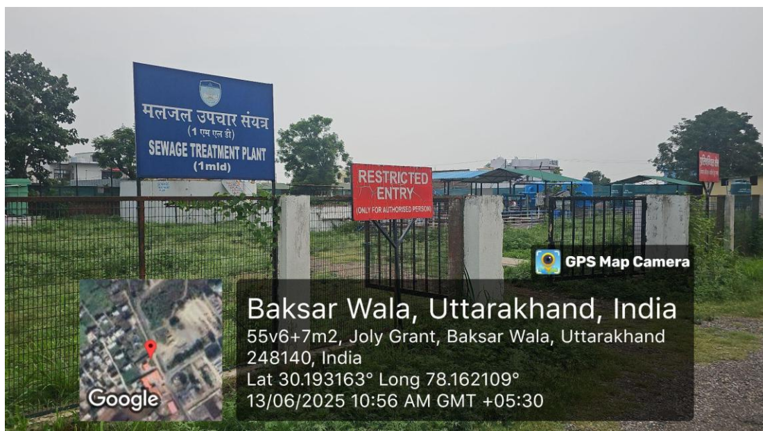
Sewage Treatment Plant at the University
