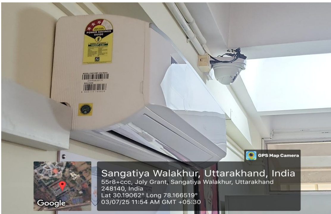
Energy Efficient split inverter air conditioners
