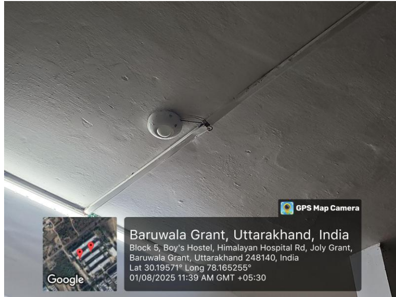
Motion based sensor lights at the Block 5, Boys Hostel, SRHU
