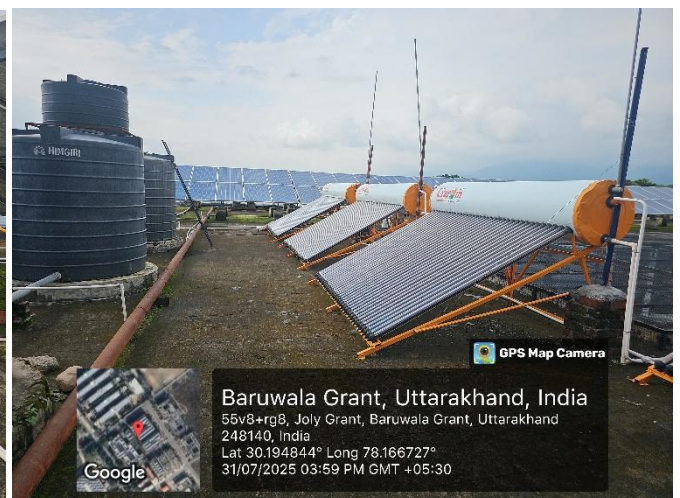
Solar water Heater installed at the rooftop of working women hostel
