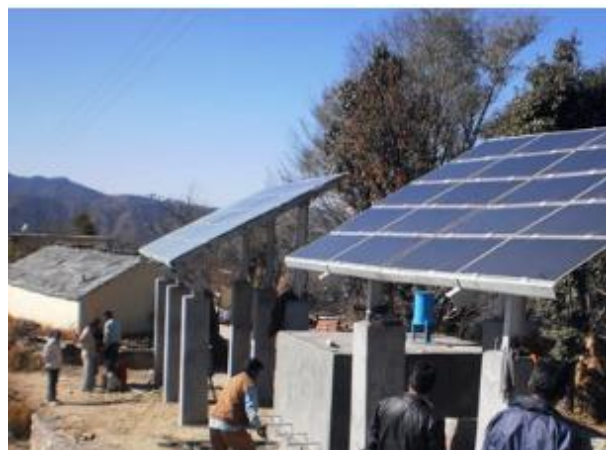
Solar power system installation in Rural Uttarakhand
