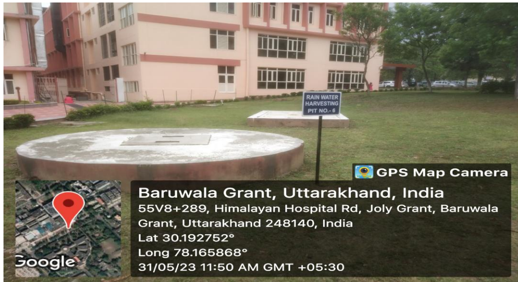
Rain Water Harvesting pit
