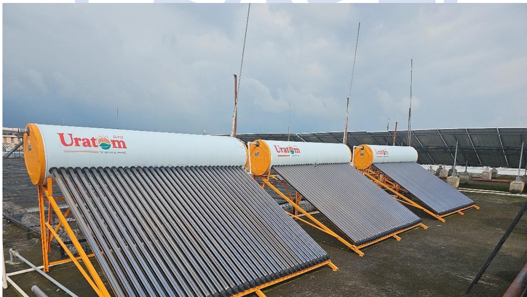
Solar water-heating systems in hostels and hospital facilities further reduce electrical demand
