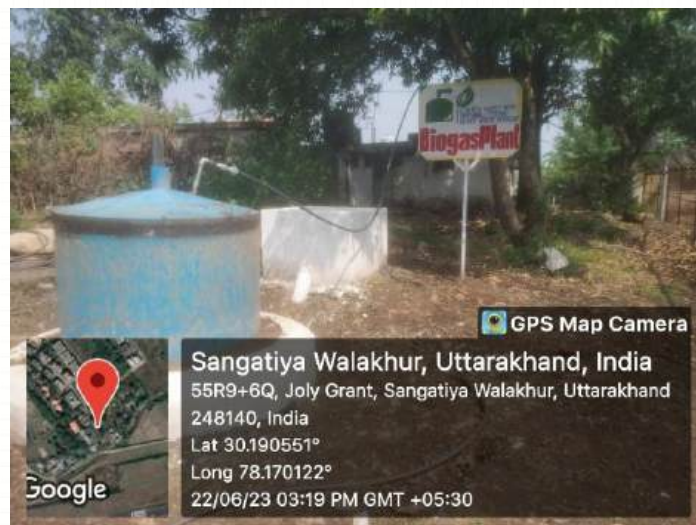
Biogas Plant at SRHU campus near University guest house
