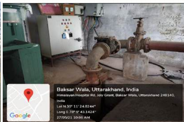
Distribution pipe from the tubewell to underground tank and the distribution system from Tubewell no.2
