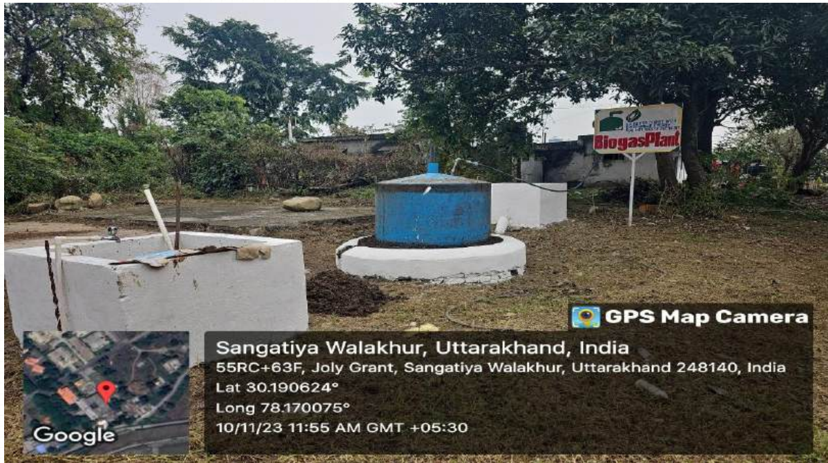
Biogas Plant near University Guest House
