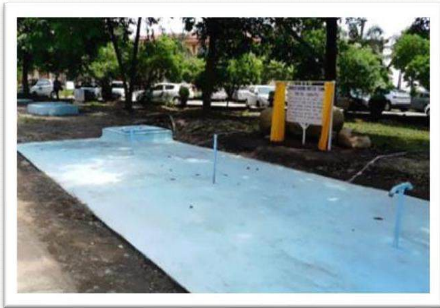
Underground water storage tank
