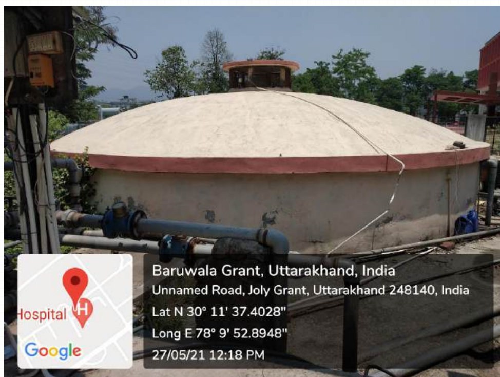
Underground water tanks (Tube well Chowk- 150 KL and behind the main Hospital building- 175 KL)
