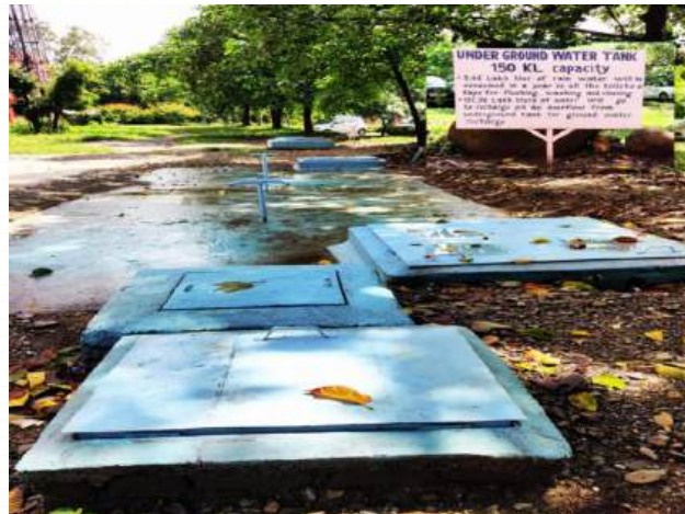
Underground RWH tank (capacity 150 KL)
