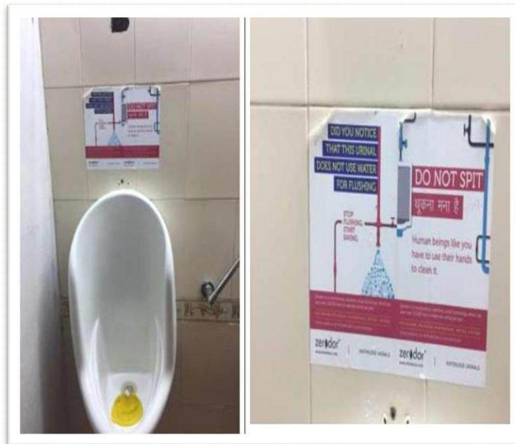
Installation of waterless urinals to save water and energy
