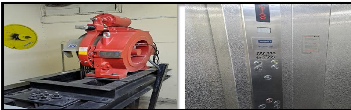
Figure 4-16 Johnson lift &amp; motor.
