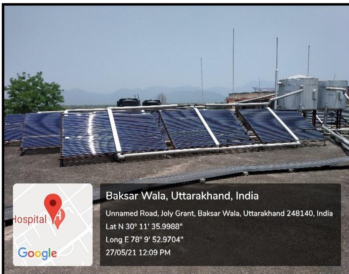
Figure 4-6 Solar water heating system
