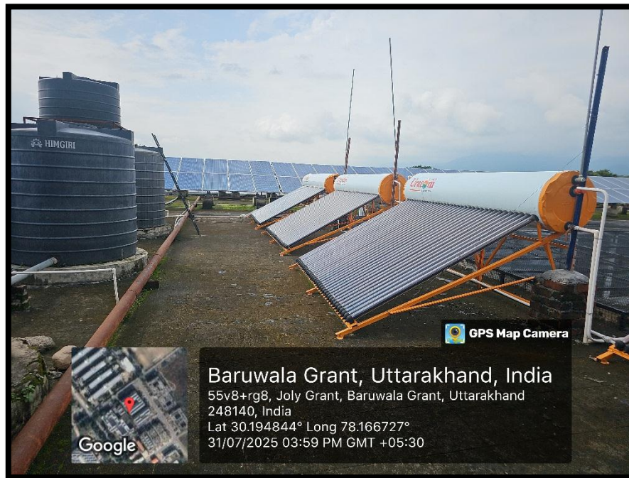
Figure 7.4. Solar water heater system within the campus
