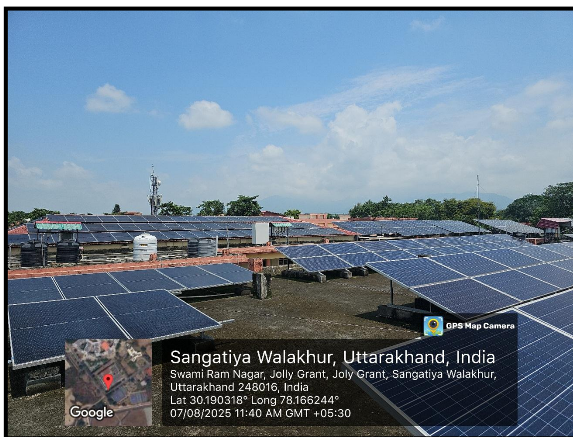
Figure 7.3. Solar Power System installed at SRHU (2.5 MW)
