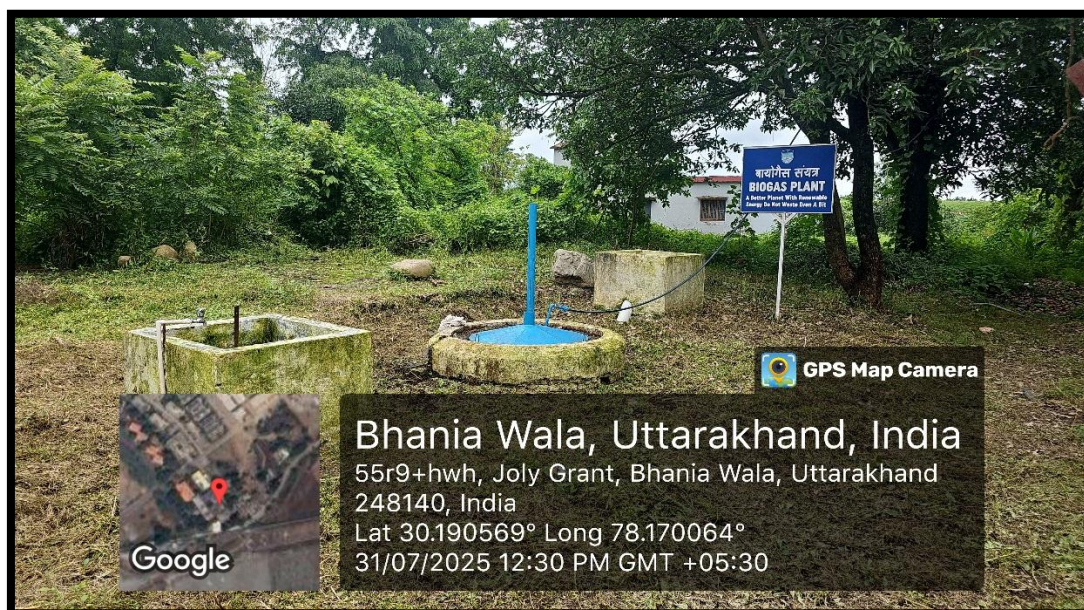
Figure 7.6. Bio-gas Plant of capacity 4 cum/day
