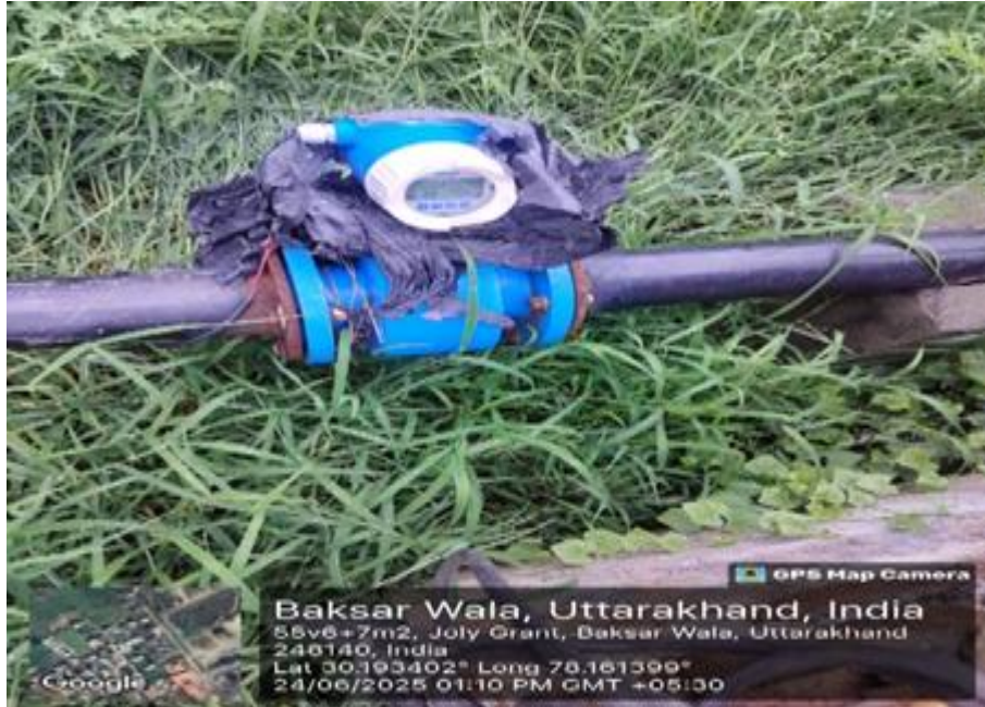
Water flow meter monitoring system from water inlet and outlet
