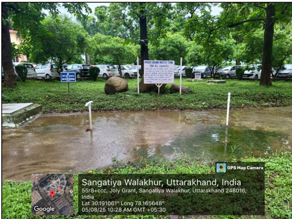
Underground water tank at SRHU
