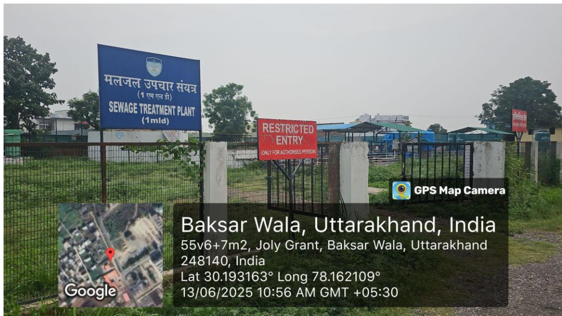
Sewage Treatment Plant at the University
