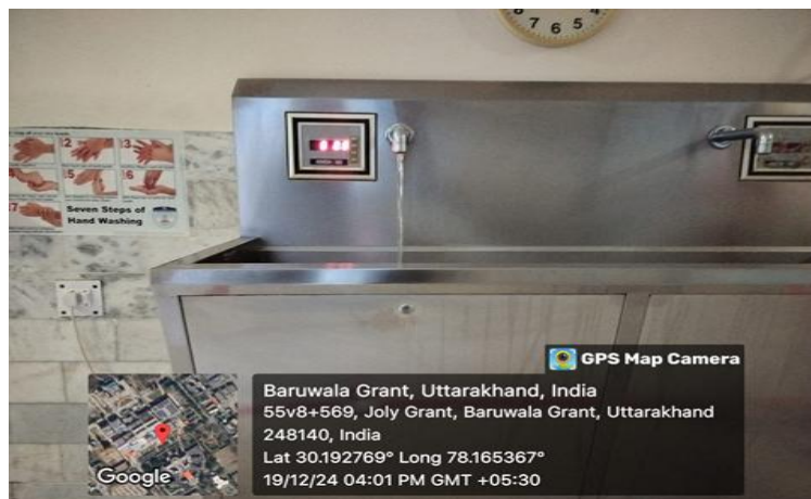
Sensor activated scrub station aiding in water conservation
