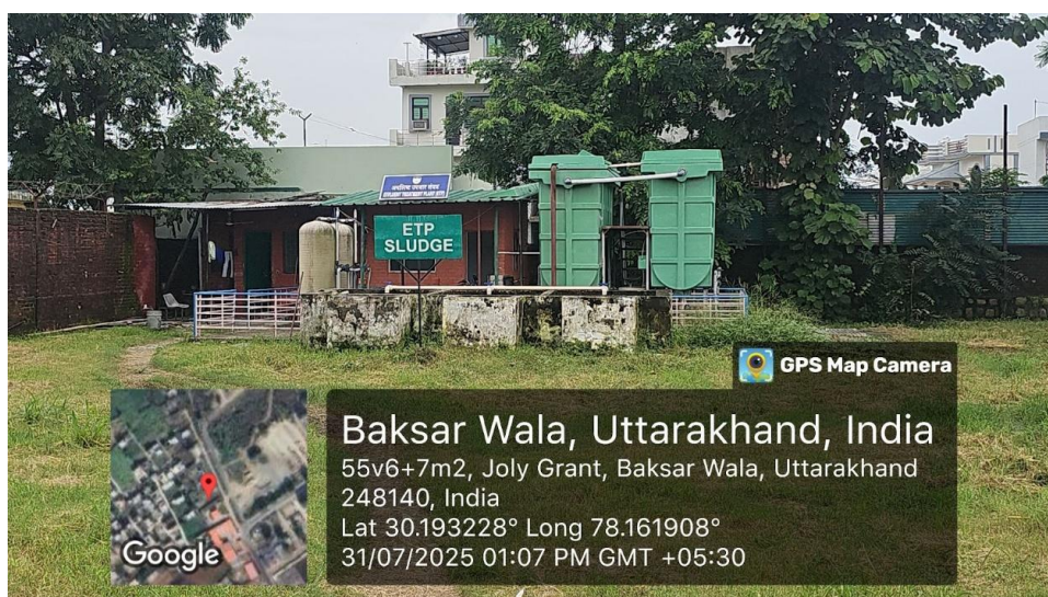
Effluent Treatment Plant at SRHU for treatment of clinical and laboratory effluent
