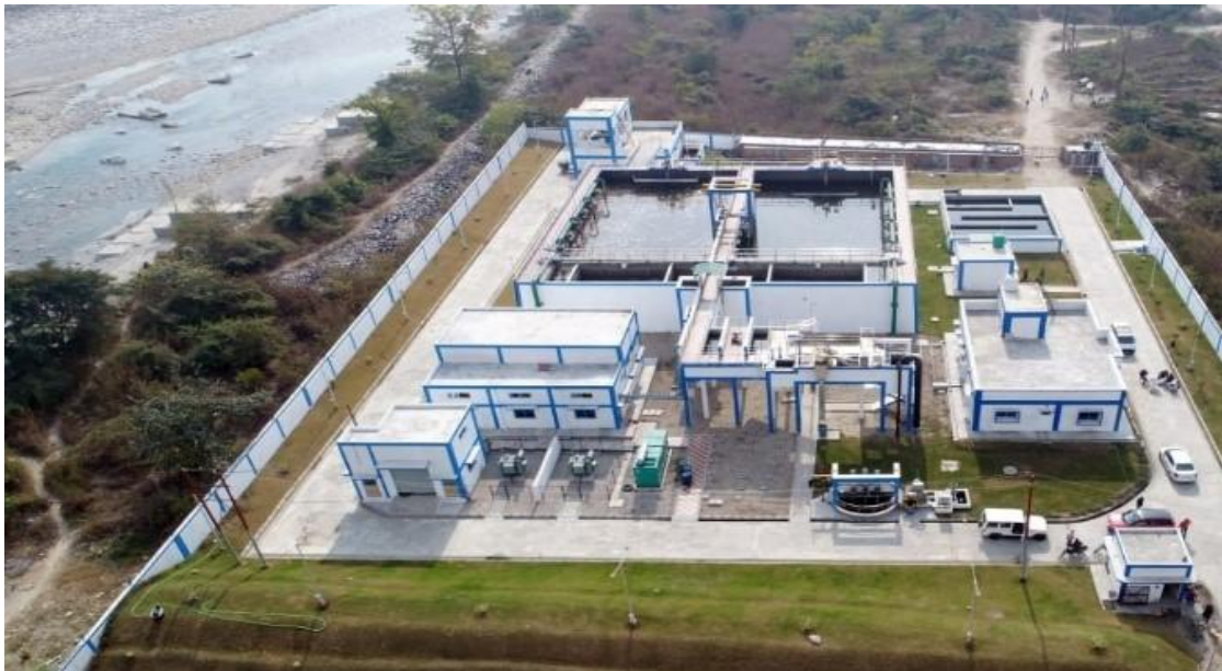
STP under Namami Gange Initiative
