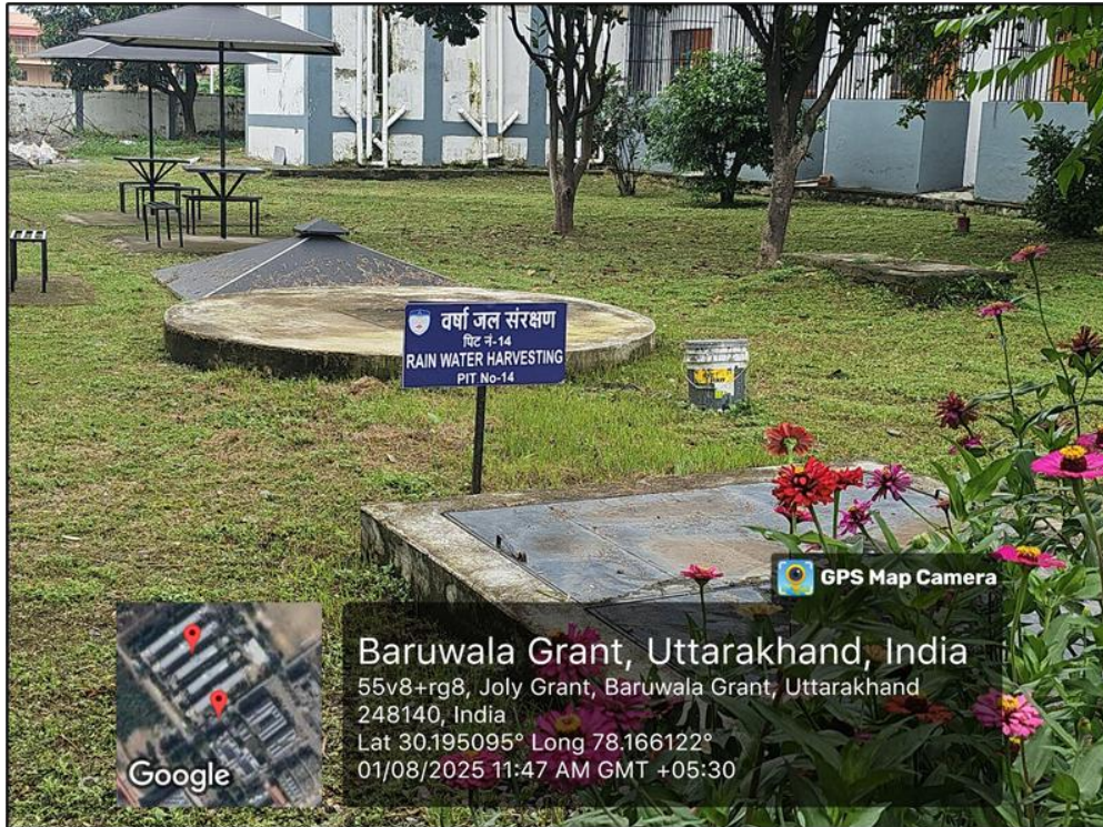
Rainwater harvesting pit near MBBS girls hostel
