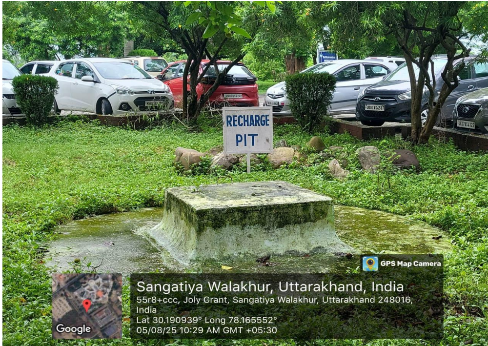
Recharge Pit near University Office
