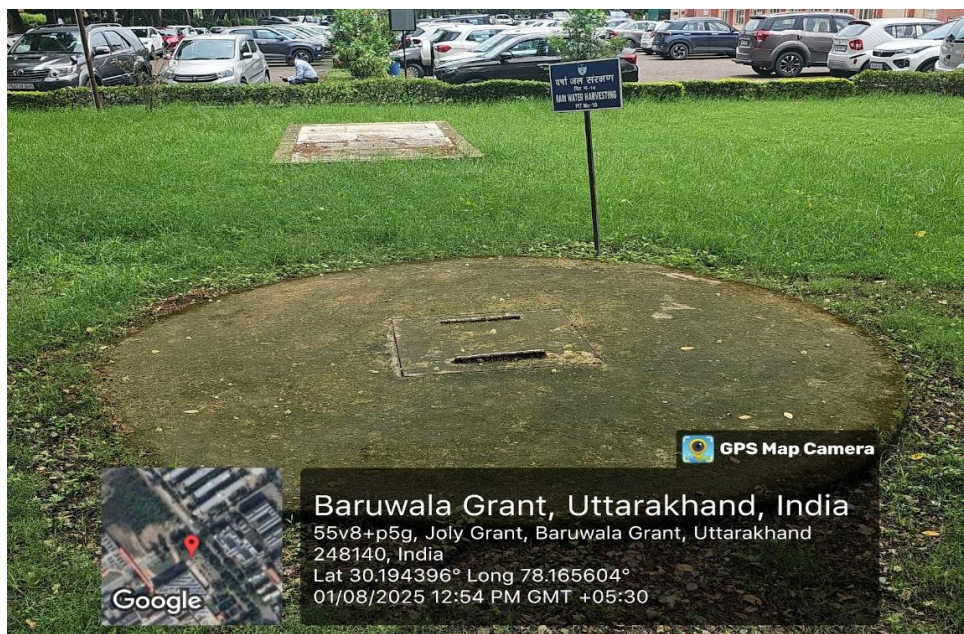
Rainwater harvesting pit at SRHU near New Block
